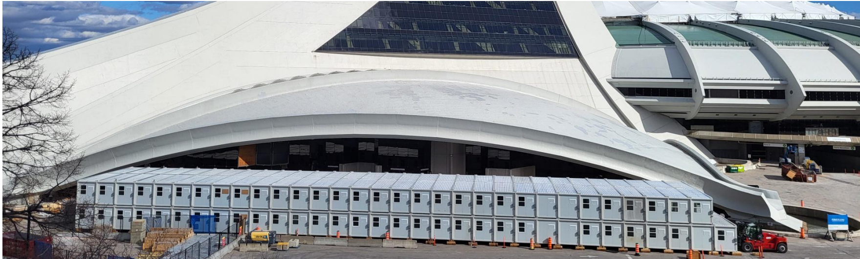
132 FLEX units in use during an Olympic stadium project in Montreal.
