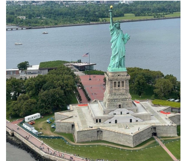
WillScot supports repairs at the Statue of Liberty...
